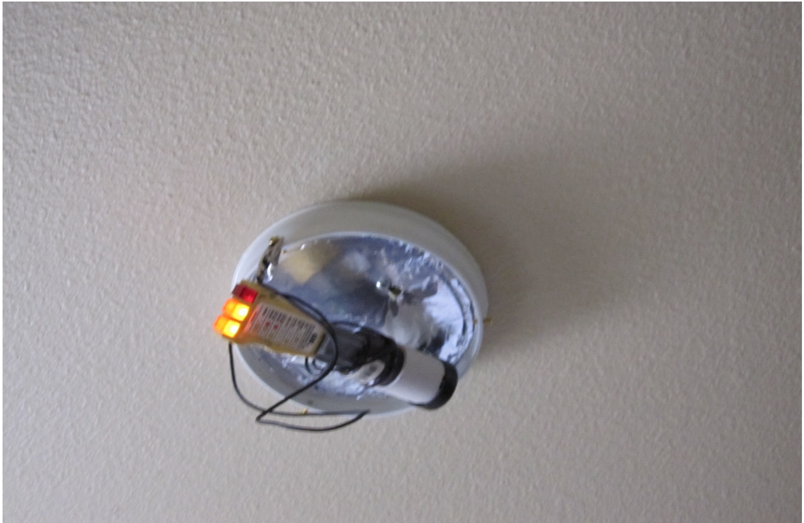
Light Fixture Test with Adaptor and ground wire
