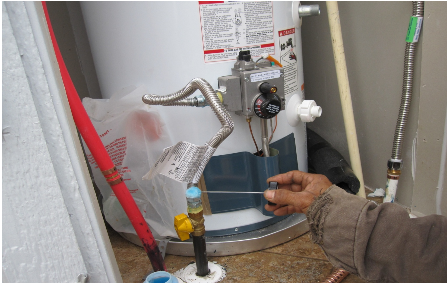
Checking for leaks on flex line
